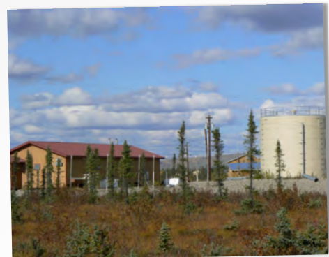
Community washeteria and water tank.
