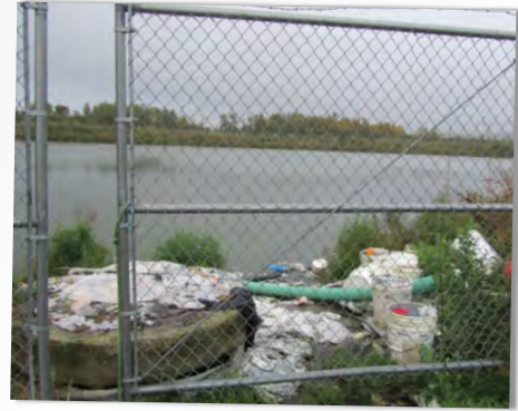
Improving lagoon monitoring & maintenance will keep the systems healthier & working more efficiently.
