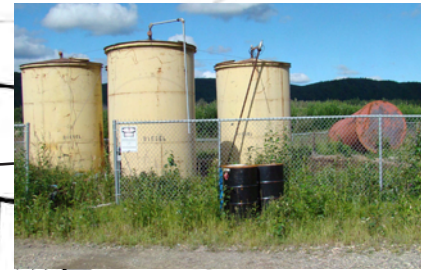
Former Tank Farm tanks
