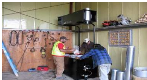
Setting up a used oil burner in Tanana.
