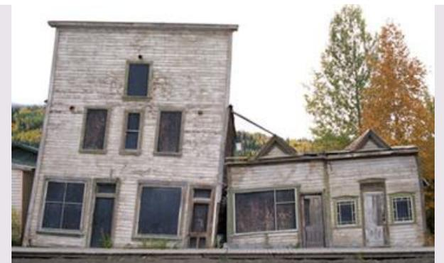
"Drunken Houses" that are falling over due to permafrost thaw
