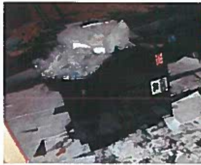
This used oil tank was not elevated or secure.
