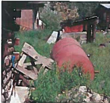
Oil spill and loss of heating capacity occurred when this unsecured tank fell from wood cradle.
