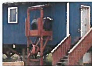
This elevated tank is protected from falling snow and ice. The diagonal wood bracing may be inadequate during a large earthquake. Steel framing connectors would add strength.
